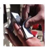
2. Attach tall ColorBracket bar mount through the Shingle Plate with (2) supplied Button Head Socket Cap Bolts Screws and (2) 1/4-20 Serrated Flange Hex Lock Nuts. The lock nuts should be on top. Tighten to 90-inch pounds.
