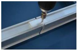
brackets, as long as the splice connectors are properly installed with 1 Tek screw each. 2"
