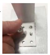
2. Carefully lift or remove roofing shingle and attach the Shingle Plate to the deck with (4) Stainless Steel Pan Head Phillips Wood Screws. Place shingle over the pan head screws leaving the bar mount exposed when the roofing shingle is placed back down over the plate.
