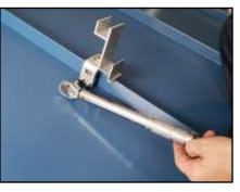
downward pressure on the assembly, torque the 3 set screws in the RoofClamp to 90 inch/lbs. Repeat this step to install a second RoofClamp/RC-2B assembly on the furthest right seam as marked in Step 2.
