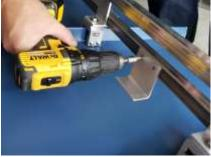
8. <u>For SnoBar</u>, butt joints should always be centered in the panel valley with no more than a 2" gap between butted ends. Some panels require the bars to be cut to obtain correct seam spacing.
