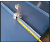
the two seams are not wider than the length of bar that you are installing. Do not place the clamps over clips whenever possible to avoid restricting the thermal expansion of the panels.
