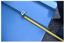
3. Set the first SnoBar Clamp onto the furthest left seam of the bar section at your 1st pencil mark. Hand tighten the set screws to the seam, making sure the clamp is centered and the bottom of clamp is down tight to the top of the seam. The (2) holes in the bar receiver section of the SnoBar Clamp should be facing upslope when properly
