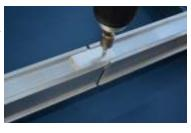
side the ColorBrackets, as long as splice connectors are properly installed with 1 Tek screw each. ColorStrips can be installed on the face of the ColorBar and in front slot of the Tall ColorBracket.
