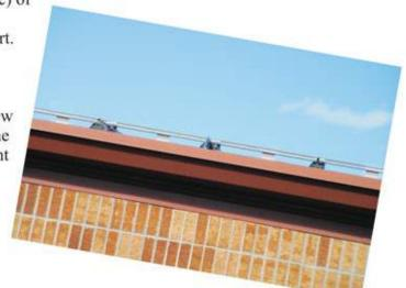
The WINDBAR system has been factory tested to the ASTM E-1592 on several types of panels (call for a test report), as well as field tested, having been used on a metal roof surviving a hurricane in an area where other roofs blew off.
